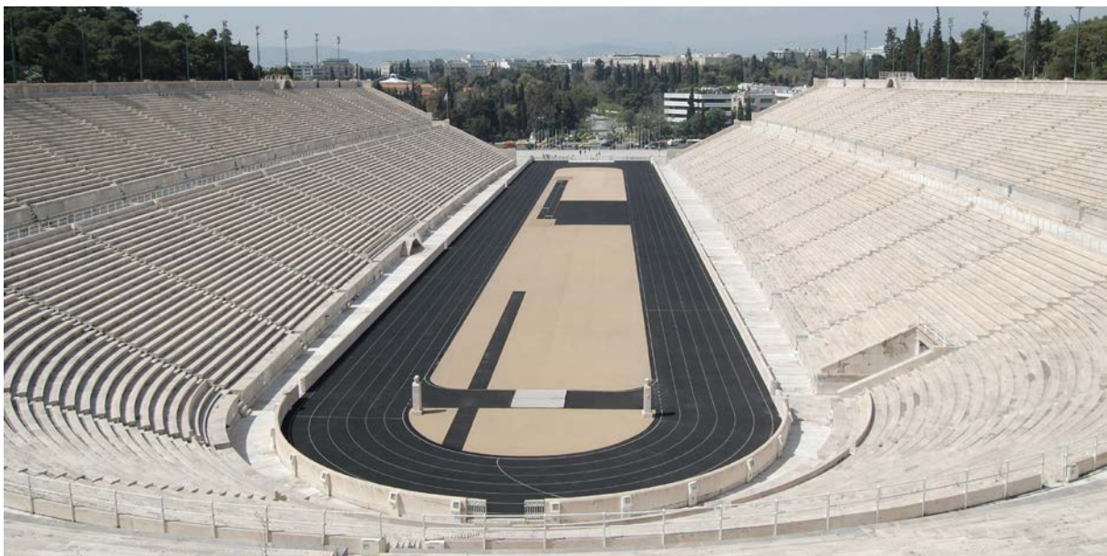
Panathenaic Stadium in Athens, Greece. Built in 330 BC and refurbished for the first modern Olympic games in 1896 AC, it is the only stadium made entirely of marble, hence the name Kallimármaro (meaning “beautifully marbled” in Greek). Like other early stadiums, the Kallimármaro was constructed between two hills to provide for natural seating tiers.
